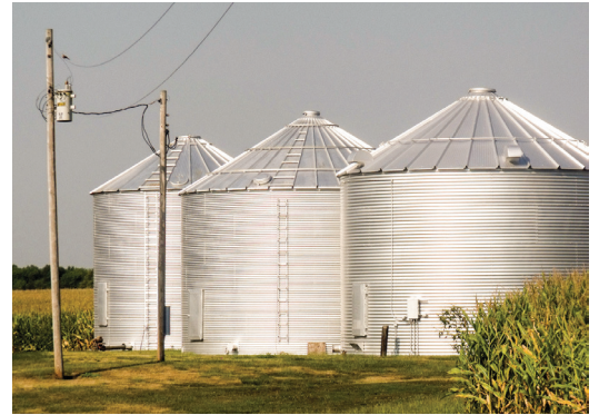
Building a structure too close to overhead power lines can create an electric shock danger during and after construction.
